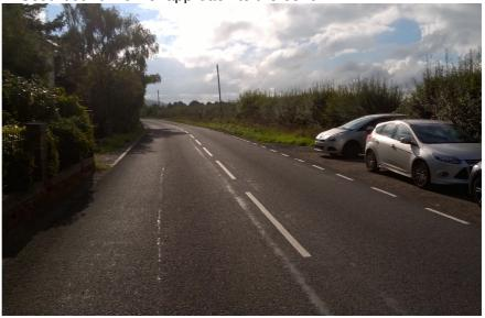
The proposed surface treatment and the removal of the centre lines, both intended to visually narrow the road, encourage vehicles to drive in the centre of the carriageway. There is a risk of head-on or side swipe collisions as vehicles enter the bend. The removal of the centre lines also increases the risk of vehicles cutting the across the curve of the bend, entering the opposing carriageway and being involved in a collision with a vehicle travelling in the opposite direction
