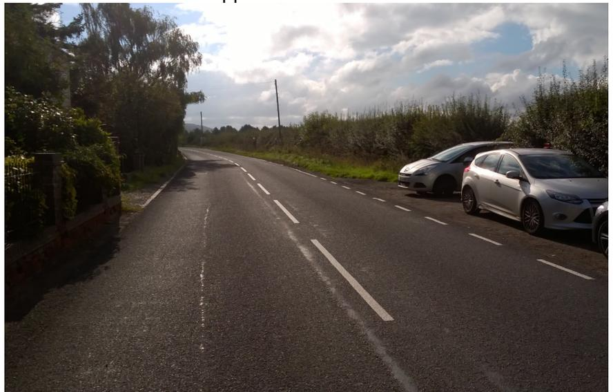
The proposed surface treatment and the removal of the centre lines, both intended to visually narrow the road, encourage vehicles to drive in the centre of the carriageway. There is a risk of head-on or side swipe collisions as vehicles enter the bend. The removal of the centre lines also increases the risk of vehicles cutting across the curve of the bend, entering the opposing carriageway and being involved in a collision with a vehicle travelling in the opposite direction.
